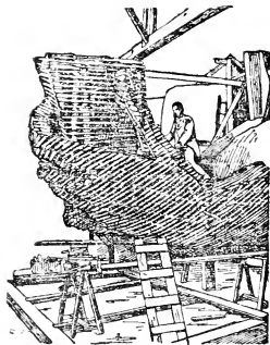
Wooden frame-work and process of modelling the left hand of the statue in plaster.
