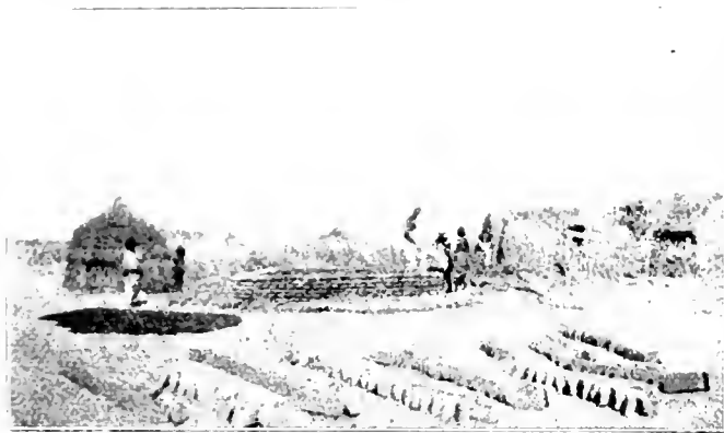
FIG. 1.—Building a Square Brick Hut. The bricks in the foreground are baking in the sun.
