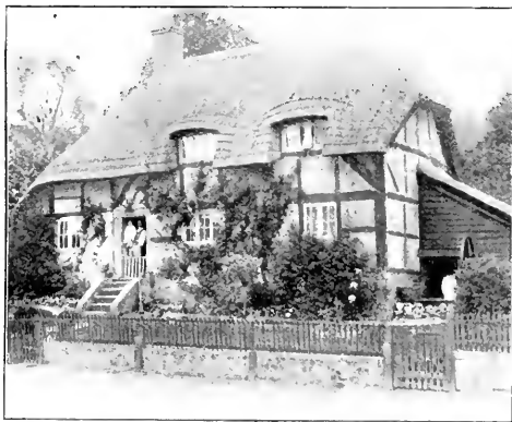
Cottages in Selborne Street, raised above the level of the road, which has been lowered by the "fretting down of ages," as in the case of many of the hollow lanes around.
