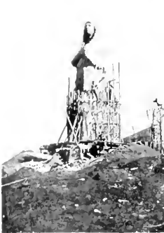
FIGURE 186. In course of erection.
