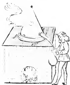
FIGURE 481. The "Roulette" still Condenser.
