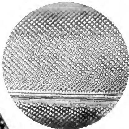
FIGURE 386. The layer underneath, showing the cause of the patches above.
