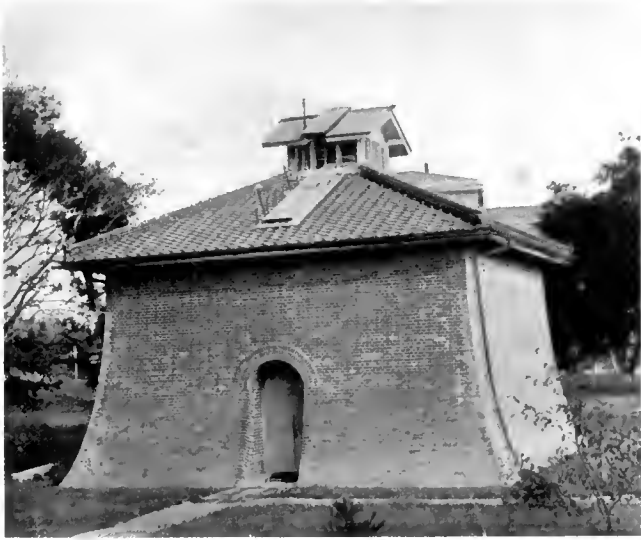
FIGURE 153. The Earthquake-proof Building erected in the grounds of the Imperial University, Tokyo.
