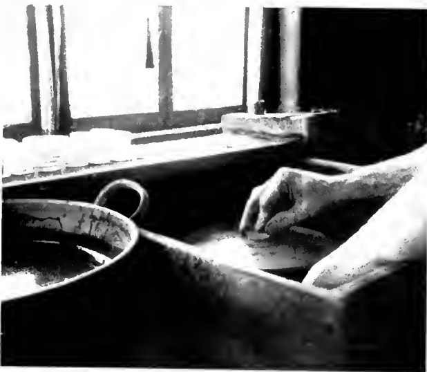
FIGURE 254. Roughing or getting the lenses into shape for polishing.
