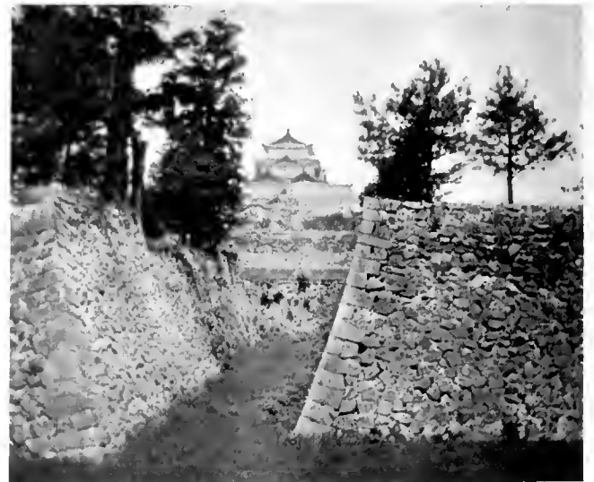
FIGURE 154. Nagoya Castle, one of the "sights of Japan." The walls are of parabolic sections, to give stability against earthquakes.
