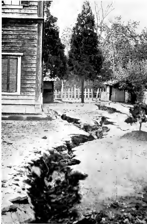
FIGURE 152. Earthquake Crack three feet wide, made during the great earthquake in the Yamogata prefecture (North Japan).
