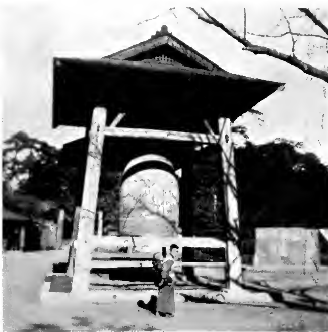
FIGURE 156. A Japanese bell-tower, wherein the suspended bell acts as a safeguard against earthquakes.
