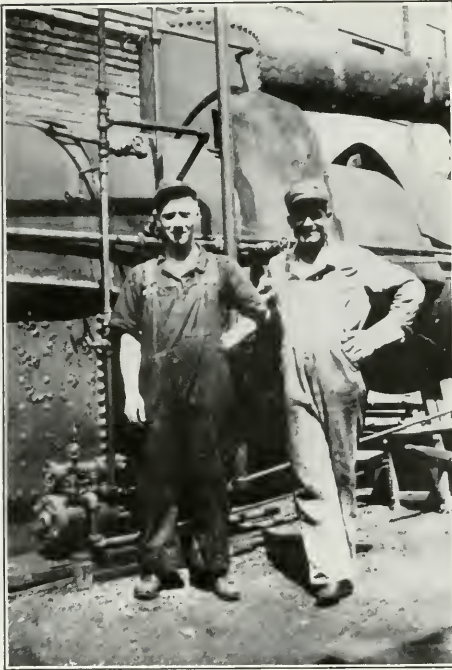
ALLIE YAHN AND FRANK GRACE With "Myrtle," the temporary boiler
