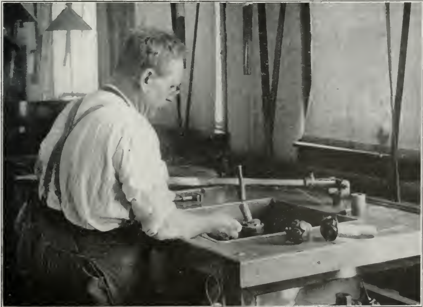
MOTOR DRIVEN MACHINE FOR ROUGH GRINDING
