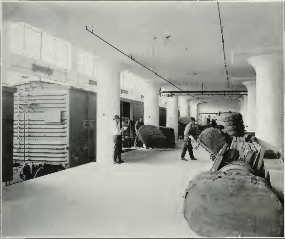
ROOM FOR SIX FREIGHT CARS AT ONE TIME
