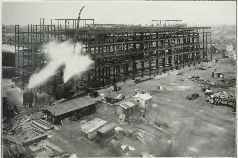
FRAMEWORK OF BUILDING 52, FEBRUARY 4, 1921
