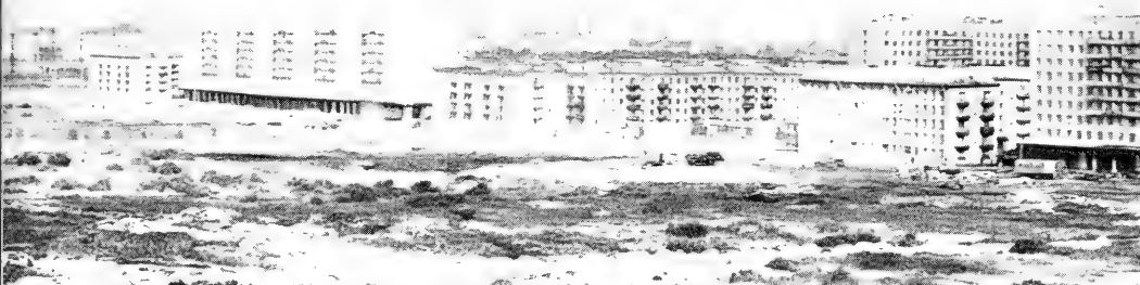
Apartment construction on south side of Leningrad behind Hotel Russia, 1964. Below, Gateway to Palace Square opposite the Winter Palace in heart of Leningrad.
