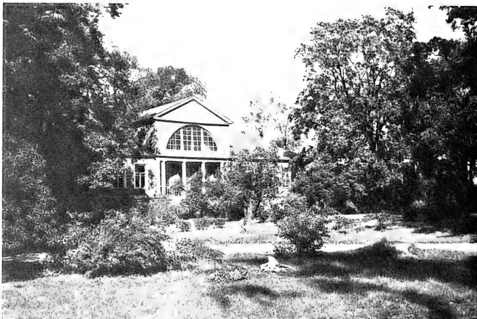
Building of Department of Geobotany, constructed in 1829.
