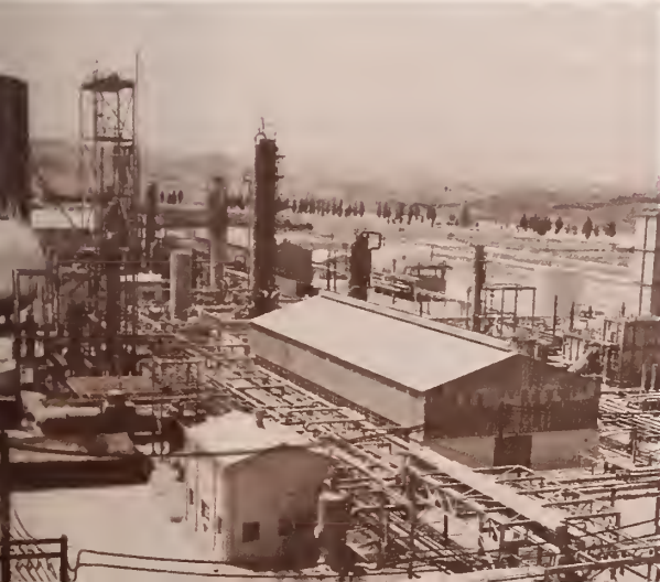
CHUNJU UREA FERTILIZER PLANT , has a capacity of 85,000 metric tons of urea fertilizer annually.
