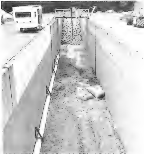
Figure 20. Relief pipe on sand bed and remains of structure I.
