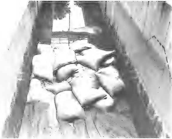
Figure 13. Front face after midtest tank draining (test I).
