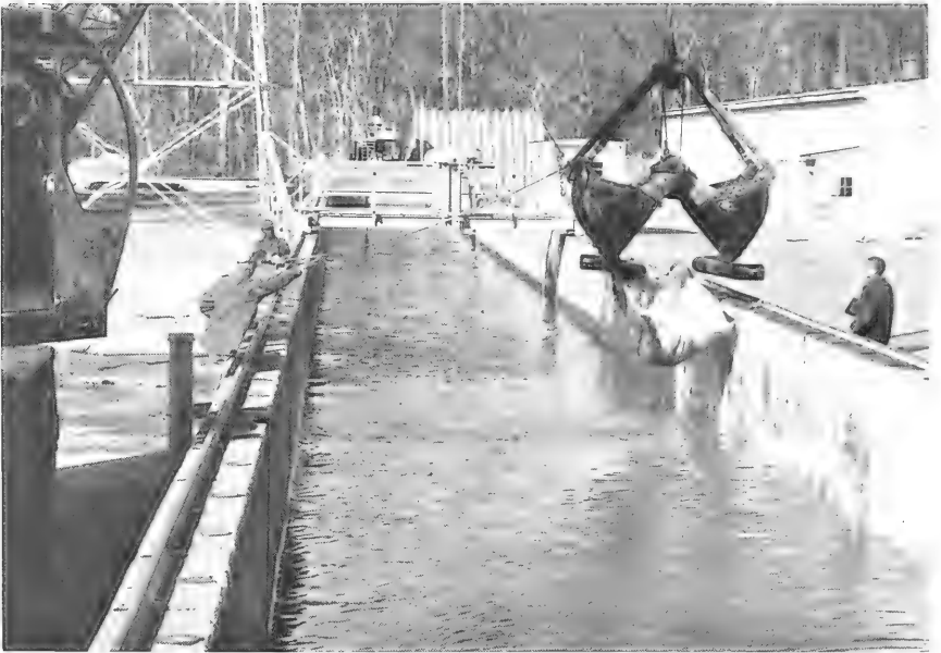
Figure 11. Placing bag.
