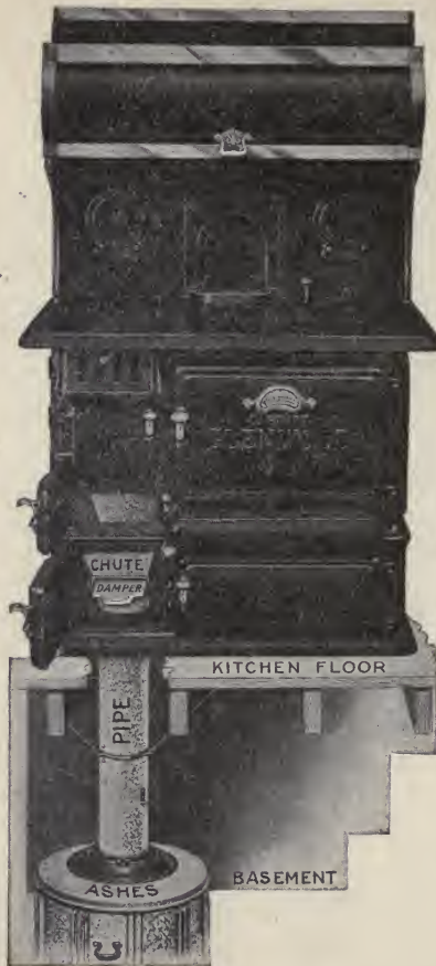
An ash-chute for the kitchen range. A decided labor saving device and should be used in every kitchen if possible.
