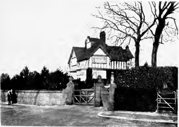
THICKETFORD (THORNTON HOUGH). [ To face p. 76. ]
