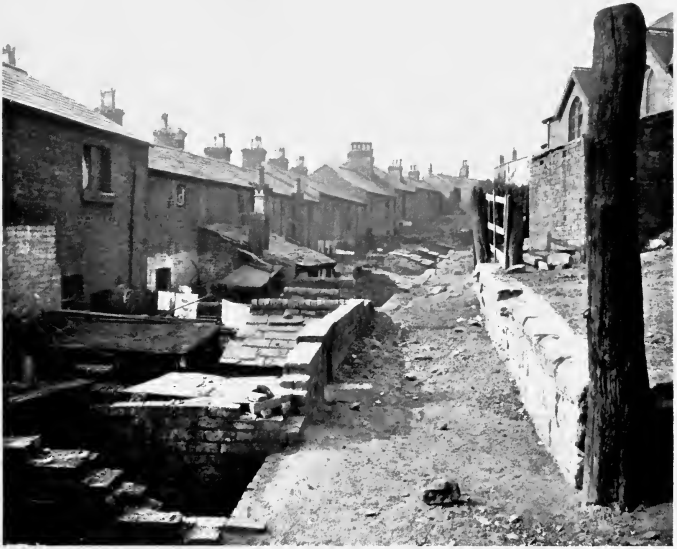
INSANITARY PROPERTY STANDING FORMERLY ON THE SITE OF THE VILLAGE.
