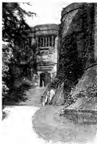
ENTRANCE TO THE CONDUIT COURT AT SKIPTON CASTLE (see page 416).
