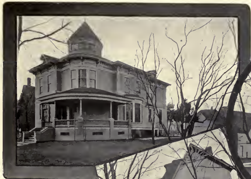
No. 19—106 South Fifth Avenue
