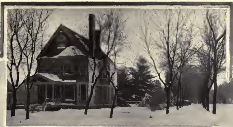
No. 9—139 South Waiola Avenue
