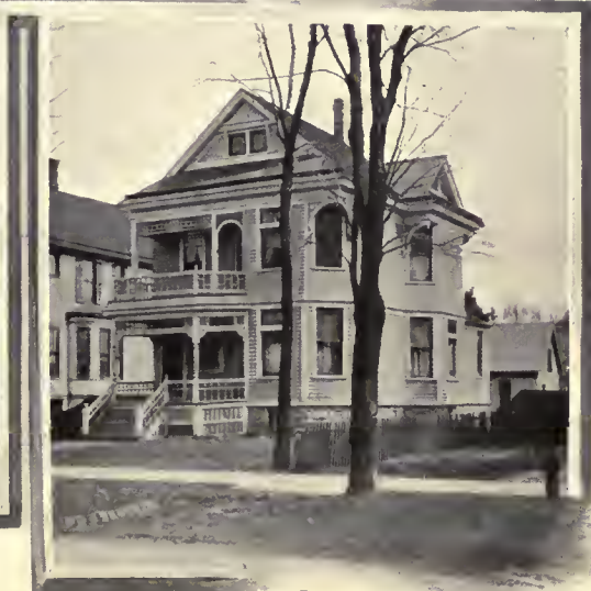
No. 11—27 South Spring Avenue
