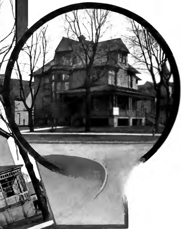
No. 18—101 North Fifth Avenue
