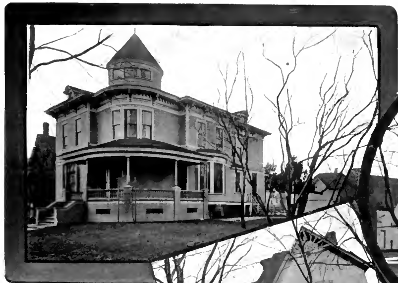
No. 19—106 South Fifth Avenue
