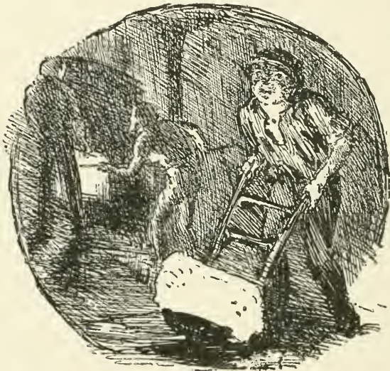
IN THE WIRE WORKS
