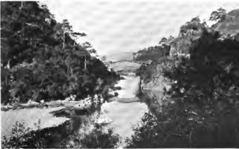
Chain and wood bridge over the Shweli (eastern branch) near Kai-t'ou
