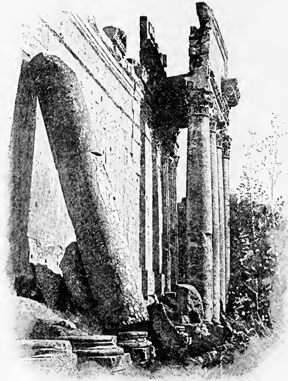
THE LEANING COLUMN ON SOUTH WALL OF THE TEMPLE.
