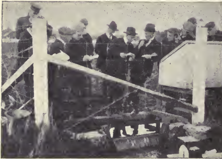
FIG. 22. Weir and drainage system outlet.
