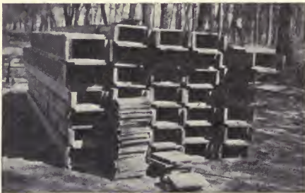
FIG. 12. Wooden box drains used at Mallet, Oregon.
