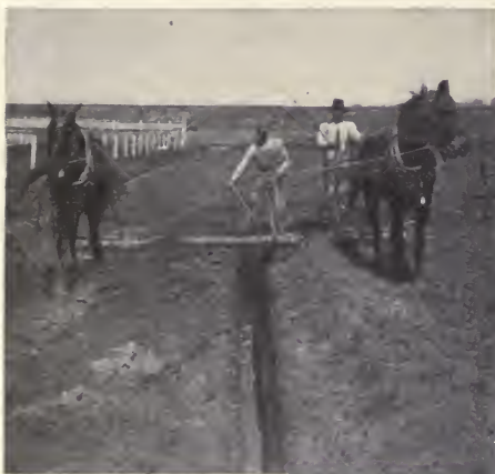
FIG. 34. Filling the tile trench with a plow. (Courtesy Iowa State College.)
