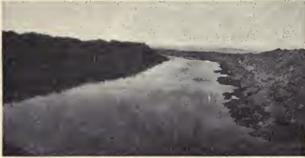
FIG. 66. A drainage canal excavated with floating dredge.
