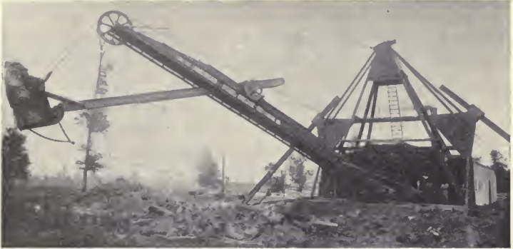
FIG. 59. A dipper dredge with bank spuds.
