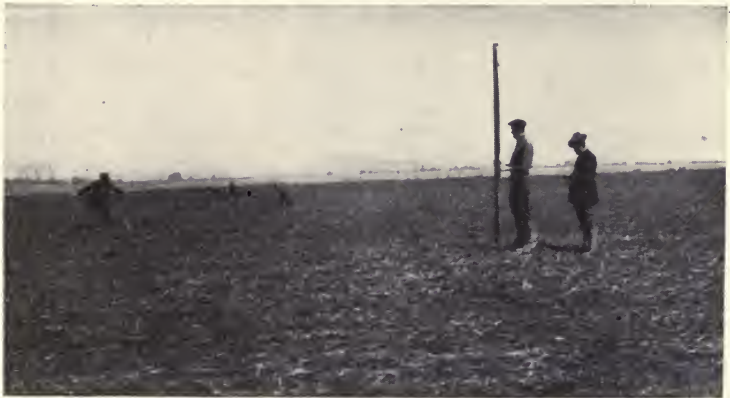
FIG. 93. Class making a survey for tile drainage.
