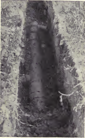
FIG. 39. View of Y-tile in trench properly laid.
