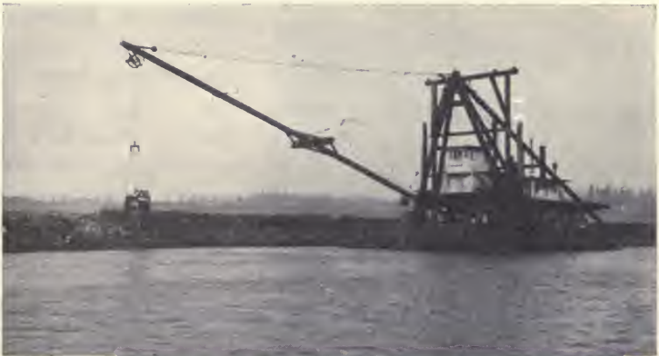
FIG. 60. A dredge with a clam-shell bucket dyking the lower Columbia river.
