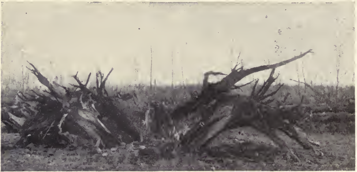
FIG. 43. A large stump cracked with dynamite before pulling. (Courtesy American Society of Agricultural Engineers.)
