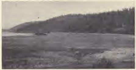
FIG. 81. Tile land in the Klamath Basin, Oregon, protected by dykes.
