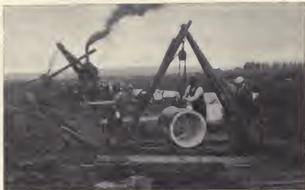
FIG. 33. Laying thirty inch tile by means of derrick and windlass.
