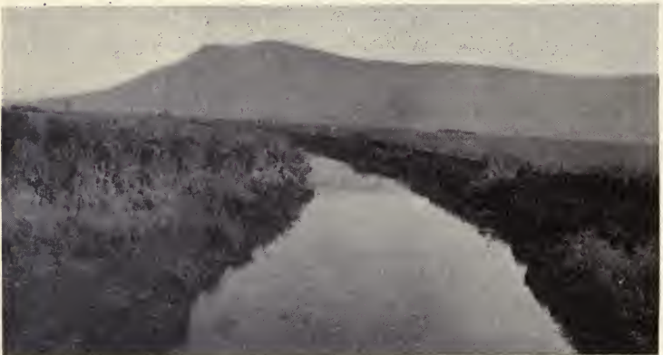
FIG. 67. Drainage canal with bank too steep and rough. Grande Ronde Valley, Oregon.
