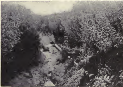
Fig. 91. Tile washed out sweet clover in use to retain banks.
