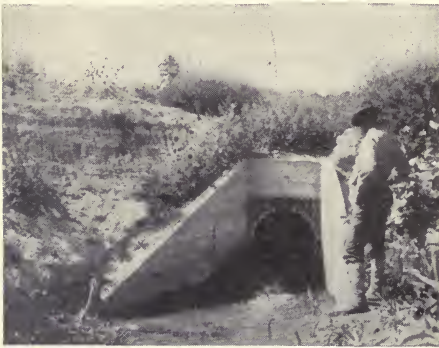
FIG. 54. Outlet bulkhead and protection. (Photograph Barr & Cunningham.)
