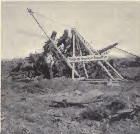
FIG. 45. A device for piling stumps. High piles burn best. (Courtesy American Society of Agricultural Engineers.)
