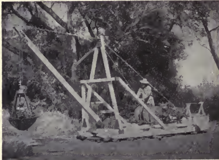
FIG. 61. A small dry land excavating outfit with orange-peel bucket.
