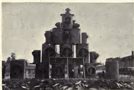
FIG. 15. Styles and forms of shale tile.
