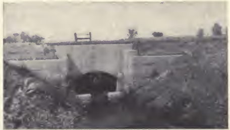
FIG. 56. A bypass for drain from Devil's Slough under Hennipin Canal in Illinois.
