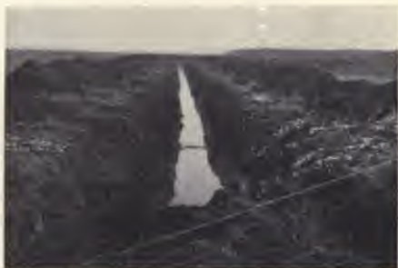
FIG. 63. Ditch excavated with the drag-line excavator shown in Fig. 62.
