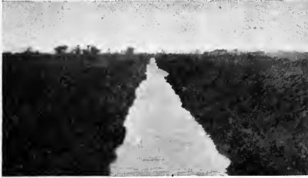
FIG. 57. Drainage outlet canal from Devil's Slough drainage district, Illinois. Represents a canal in good condition.
