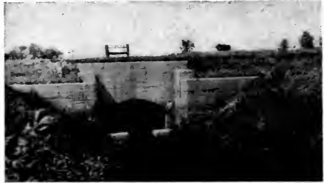
FIG. 56. A bypass for drain from Devil's Slough under Hennipin Canal in Illinois.
