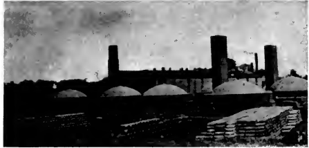
FIG. 13. Shale tile plant, Sheffield, Illinois.
