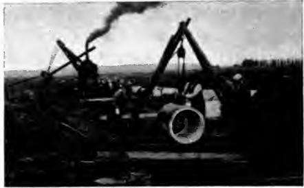
FIG. 33. Laying thirty inch tile by means of derrick and windlass.
