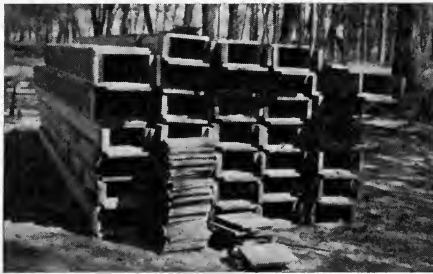
FIG. 12. Wooden box drains used at Mallet, Oregon.
