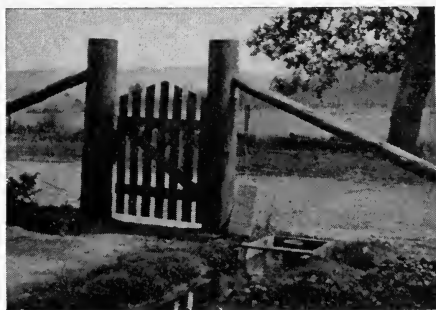
FIG. 83. Drainage water used for irrigation of lawn and garden.
