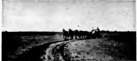
FIG. 35. Filling the tile trench with a road grader. (Courtesy Iowa State College.)
