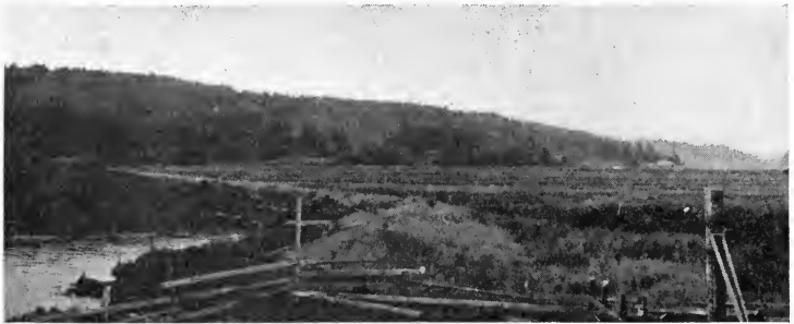
FIG. 72. Land enclosed with dyke.
