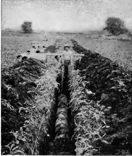
FIG. 32. Finishing trench to grade and laying tile. (Courtesy Iowa State College.)
