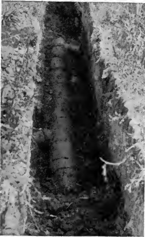
FIG. 39. View of Y-tile in trench properly laid.
