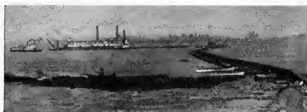
FIG. 64. Hydraulic dredge at work on lower Columbia river.
