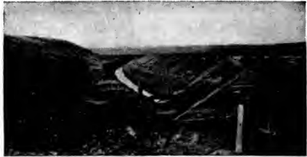
FIG. 55. Outlet ditch of Malheur Drainage District. (Photograph Barr & Cunningham).
