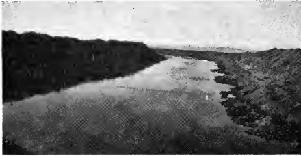
FIG. 66. A drainage canal excavated with floating dredge.
