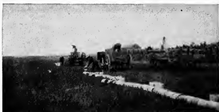
FIG. 26. Hauling and distributing tile.
