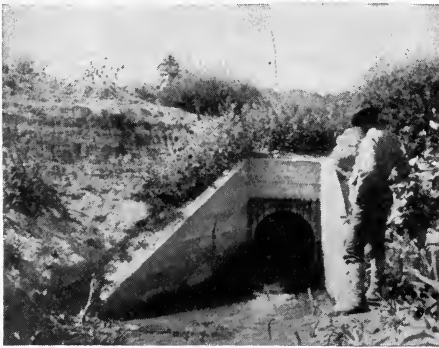
FIG. 54. Outlet bulkhead and protection. (Photograph Barr & Cunningham.)
