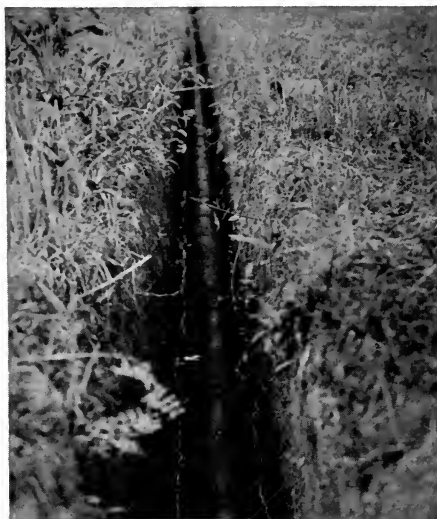
FIG. 73. Well laid tile in trench through tide land.
