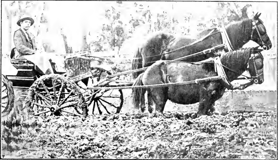
ON THE BOOLARRA-FOSTER ROAD. Since Metalled by Country Roads Board.
