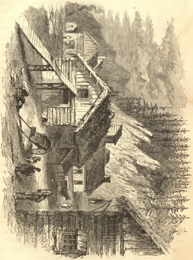
STATION-HOUSE, LOGEN VALLEY.
