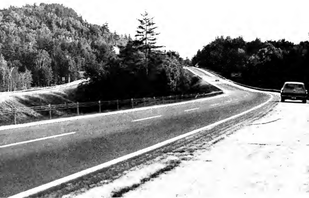
Trees between north and south lanes on this freeway in New York State reduce wind and dust activity, and lower the noise levels, as well as creating a scenic drive.
