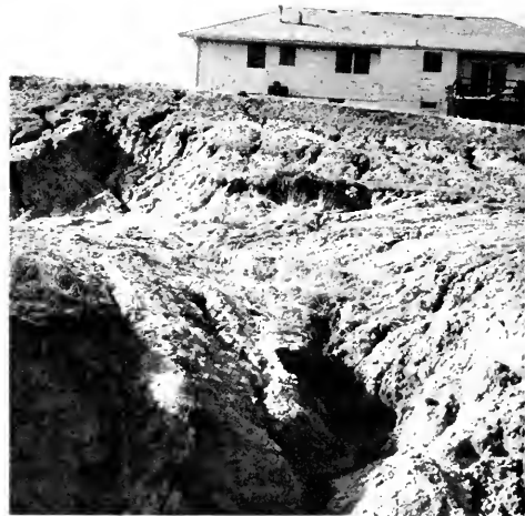
Developer of apartment complex above in Indianapolis used an excavated area for storm water storage, recreation, and for scenic value. Storm water is routed into this area and released through an outlet at a retarded rate. Right, improper disposal of surface water caused gully threatening a home in Des Moines. Below, sediment and debris fill channel of small stream where it passes through a development in Washington State.
