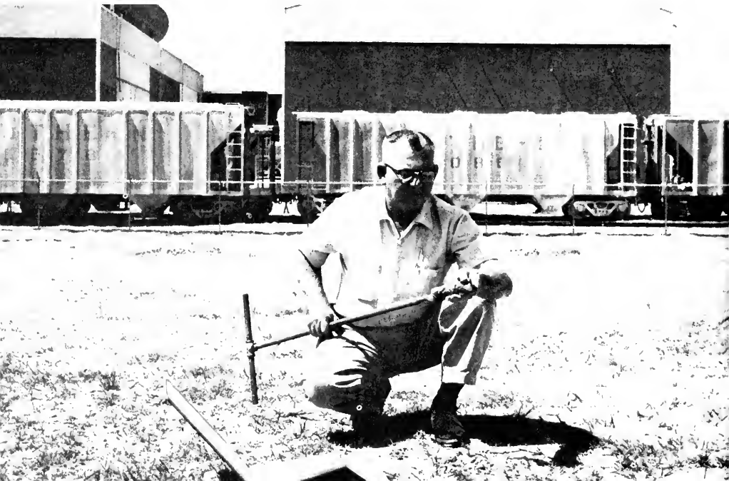
Soil scientist checks sample from an auger while mapping soils near Aiken, S. C.
