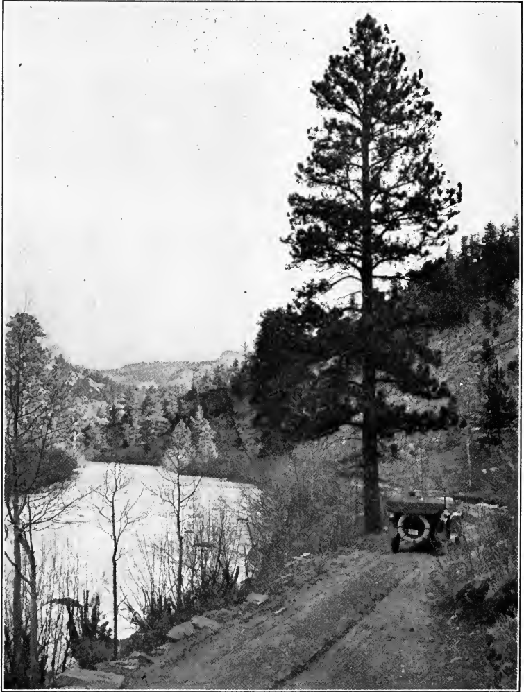
FIG. 21. — UTILIZING THE RIVER-SIDE. The bank of a river is as suitable for a road as for a railway.
