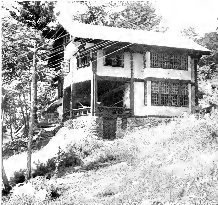
Another exception to the demand for formal treatment is the house which rises from rock formation; the third is the bungalow crouched upon sand dunes
