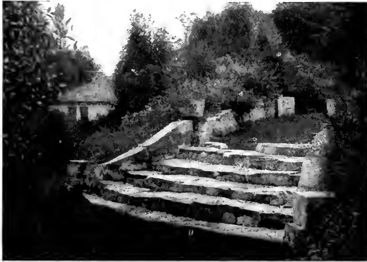
The abrupt transition from one level to another may be made the occasion for structural work that in itself adds much beauty
