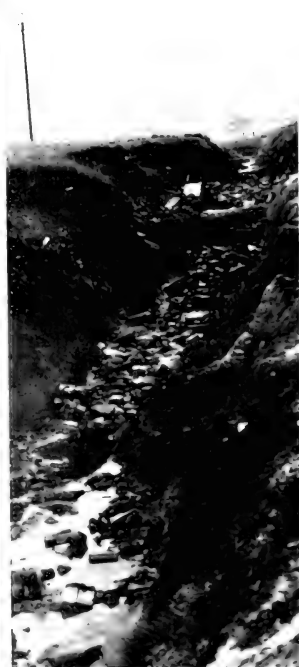
Fig. 7.3. Roddymoor reclamation site. Severe erosion on main drainage channel.
