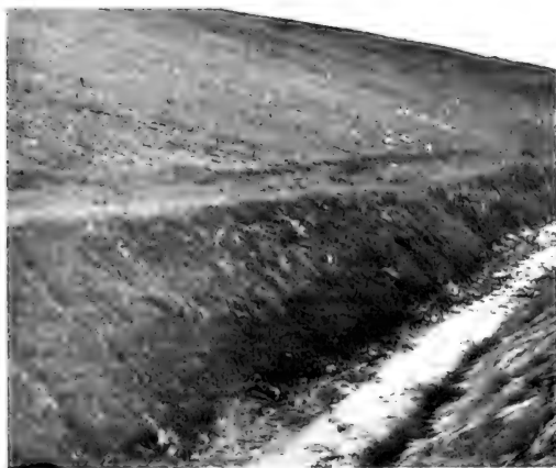
Fig.7.4 Roddymoor: Main drainage channel.
