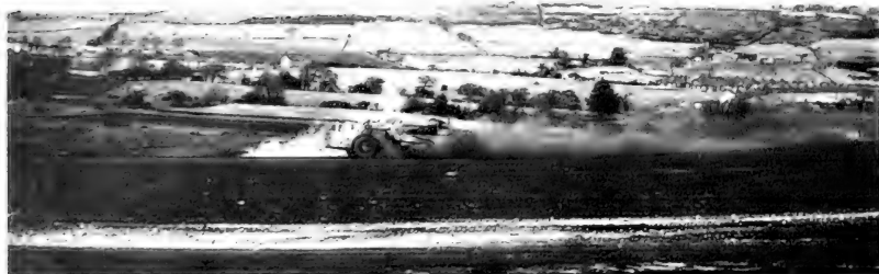
Fig. 6.4 A temporary problem with grading operations in some reclamation projects is the raising of dust clouds by earth moving machines. This illustration indicates the considerable distances over which the nuisance may occur.
