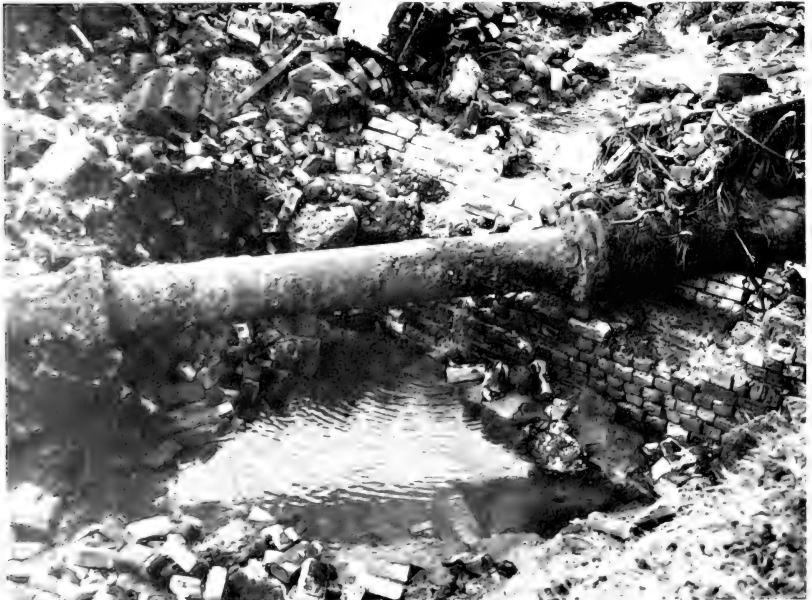
Fig 6.3 An example of the exposure of old foundations during the erosion process of a new watercourse. Recommendations for dealing with this problem are given in Chapter 7.
