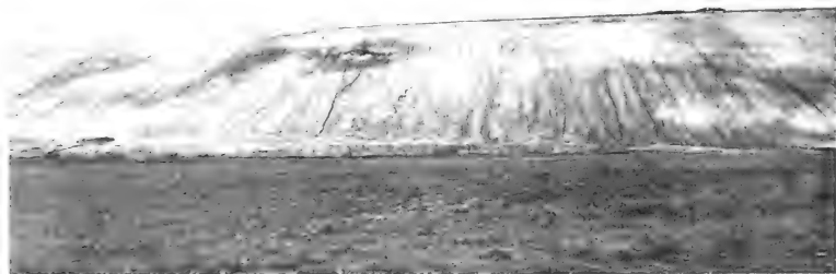
Fig. 10.3 Eroding surface on the north facing slope at Roddymoor. Rills were in evidence prior to seeding. Mulch held the slope surface until the grass became established.
