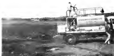
Fig. 10.2 Hydroseeding without mulch of a shallow gradient area on ash over building foundations. CP2 mixture was used. This method may have application where conventional seeding cannot be undertaken because underlying foundations would prevent cultivation by normal agricultural implements.
