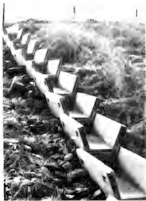
Fig.7.5 Roddymoor: Concrete flume built on steep slope.
