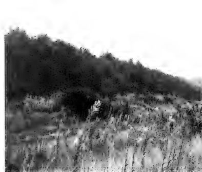
Fig 2.2 The Woodshaw Pit spoil heap in Lancashire is an early example of a reclamation technique involving planting on unaltered pit heaps (Courtesy of Lancashire County Planning Department).
