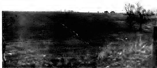
Fig.7.1 Roddymoor, Crook: Temporary open ditches to check surface water run off N.C.B. (Opencast) Site.
