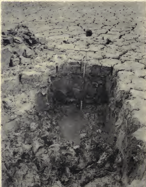
Where does soil washed from farms go? Here is one answer. In this reservoir near Columbus, Ohio, 30 inches of silt -- normally under 20 feet of water, have been collected in ten years.
