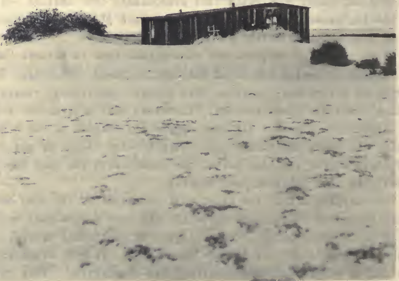
Windblown material has almost covered this farmhouse in Eastern Colorado. Salix on the left has been buried to a height of seven feet.
