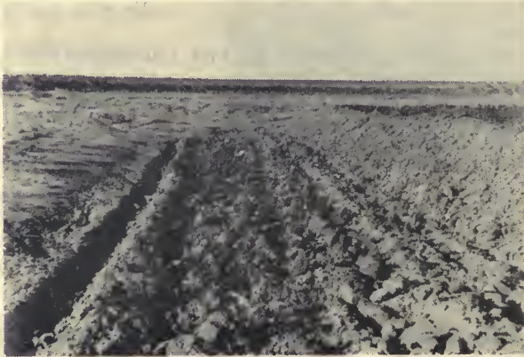
Compacted earth in terrace channel torn up with road ripper.
