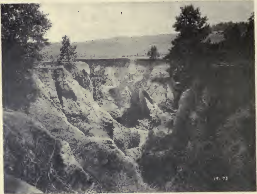
View from Hix Gully, showing laterals due to improper terrace outlets.
