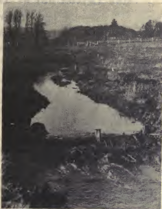
The same check dam, completed, being given a severe test.
