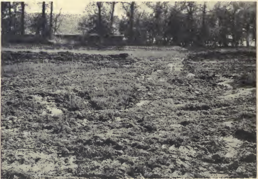
SES-1/202. Field north of home showing terrace outlet channel after terraces have been built but before any work has been done on the outlet channel. Sept. 24, 1934.
