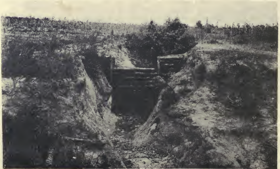
The same gully, effectively checked with an inexpensive log dam.
