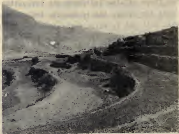
Erosion control as practiced by the Ancient Peruvians. Detail of bench terraces in the Colca Valley.
