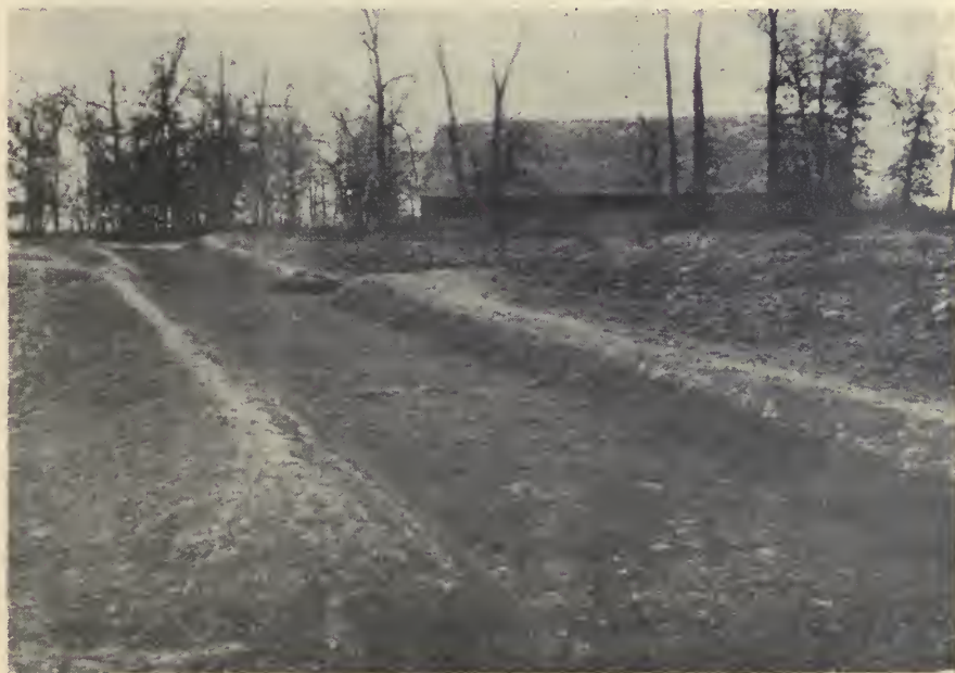
SES-1/241. Sodded terrace outlet on E. H. Johnson farm, Vernon County, Wisconsin. This is a repeat photograph of the same land in the previous picture. Oct. 15, 1934.
