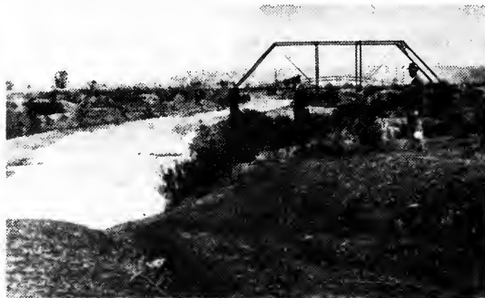
The meandering stream has left this bridge utterly useless.
