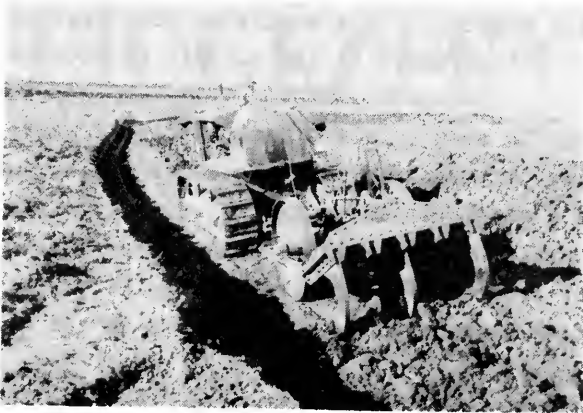
Ripper loosening compacted soil in terrace channel. Earth will be removed with a rotary fresno to build up a low place in the terrace ridge.
