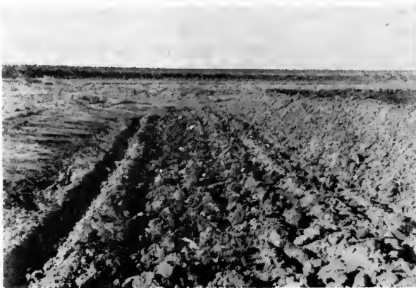
Compacted earth in terrace channel torn up with road ripper.
