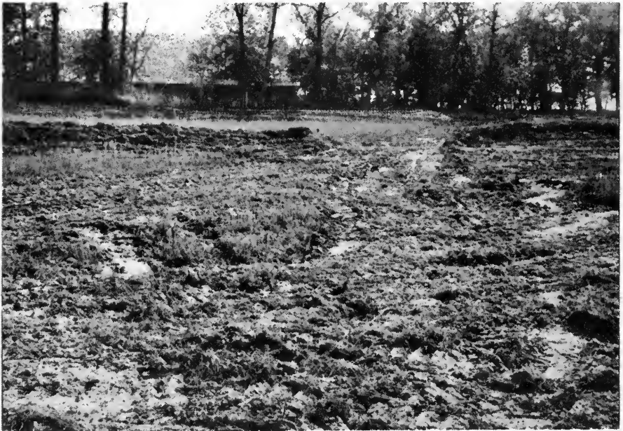
SES-1/202. Field north of home showing terrace outlet channel after terraces have been built but before any work has been done on the outlet channel. Sept. 24, 1934.
