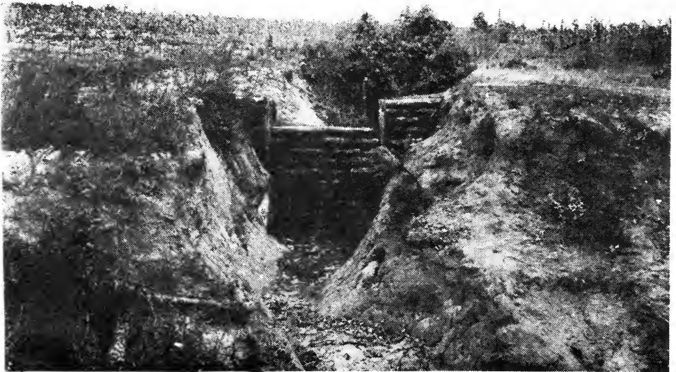
The same gully, effectively checked with an inexpensive log dam.
