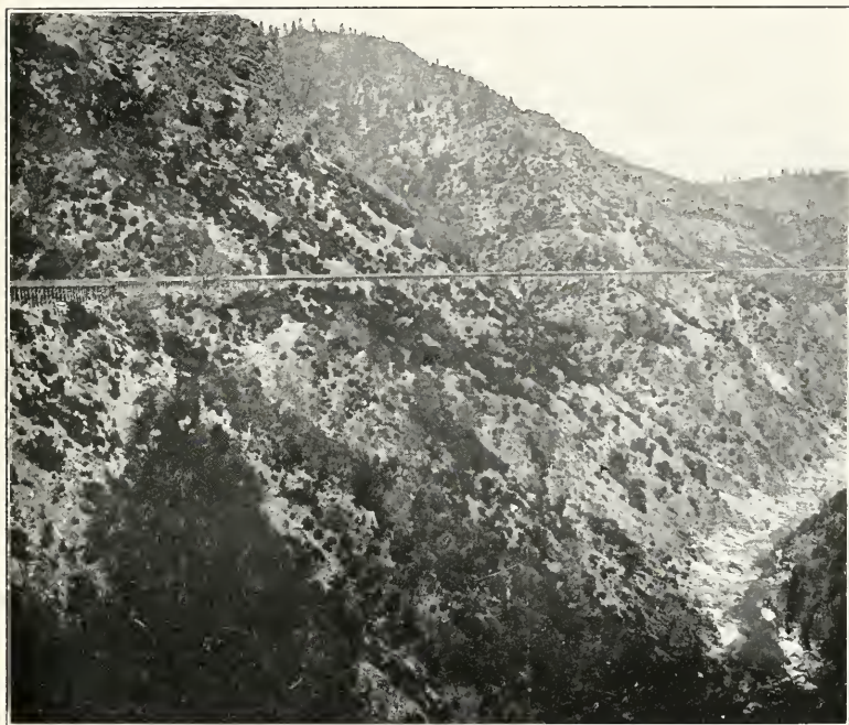
It is a great pipe line
