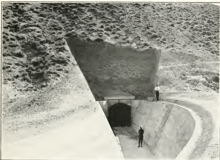
They have tunnelled through a great mountain
