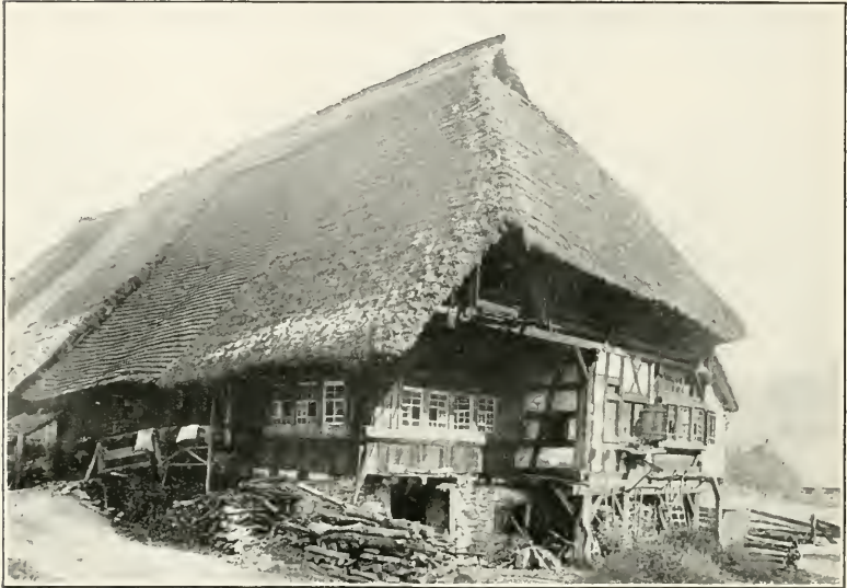
Some of the roofs are thatched with straw
