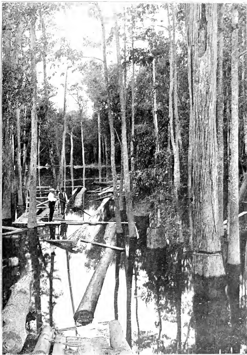
Getting cypress logs out under difficulties
