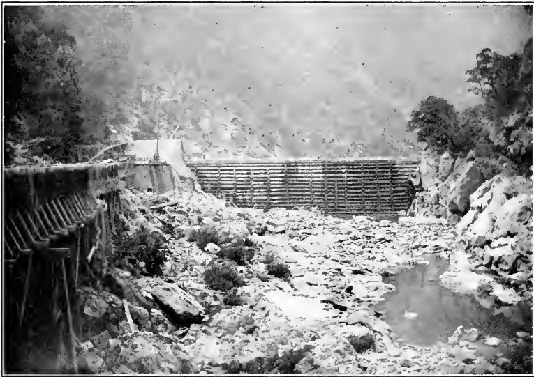
Others depend on dams for the storage of water
