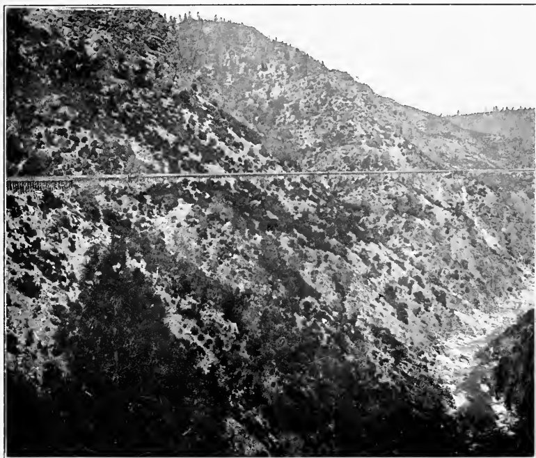
It is a great pipe line
