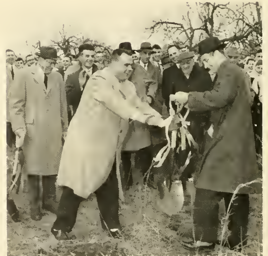
Dick helped Gil and Frank break ground for their new houses.
