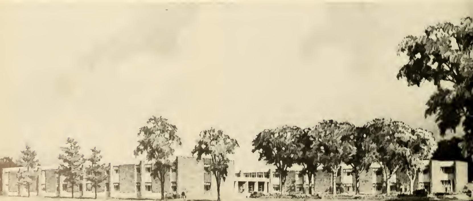
WOMEN'S DORMITORY BUILDING
