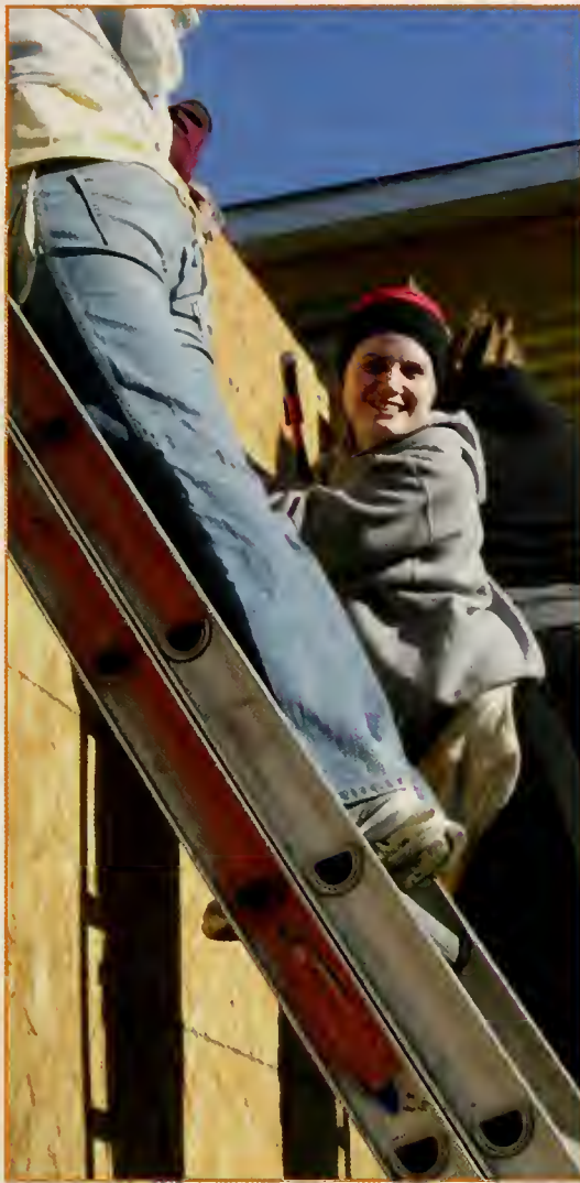
Above: Kristin Vought helps with construction work on HRT 13.
