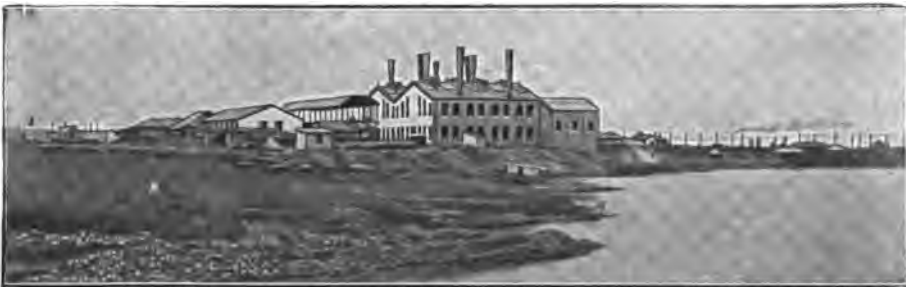
Fig. 107.—Simmerpan Power Station. General View. Management offices in foreground; the coal bunkers may be seen in front of the boiler houses.
