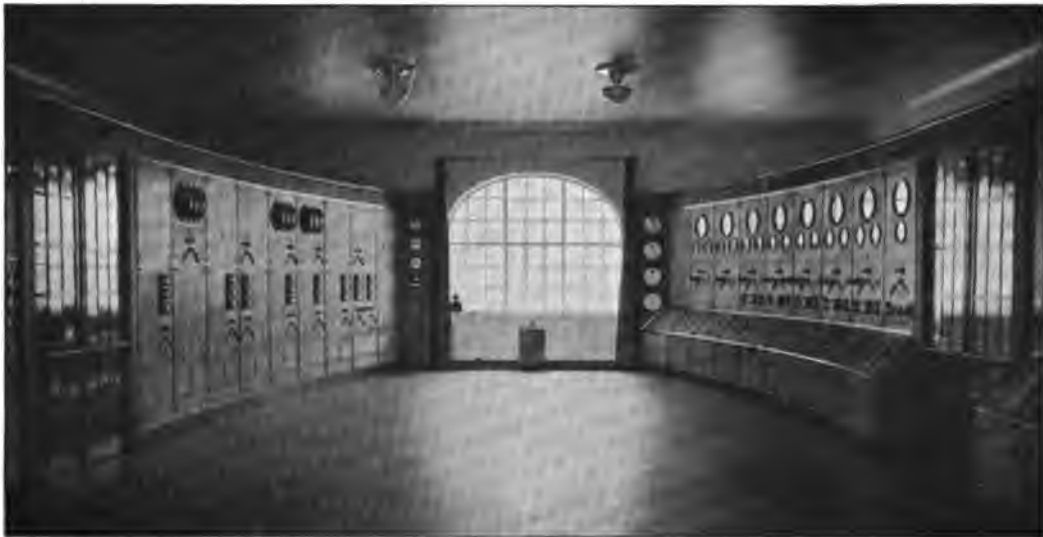
Fig. 33.—Control Board in the Switch House of the Wyhlen Electricity Works. Generator panels on the right, feeder panels on the left. Panels constructed of polished blue marble. Diagrams of connections shown on the panels by strips of polished brass.
