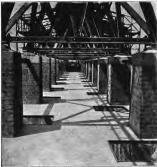
Fig. 167.—Vereeniging Power Station. Coal Store below the Railway; Pockets in the floor for filling the Bucket Conveyor.
