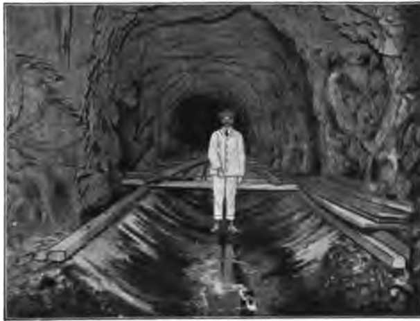
Fig. 169.—Vereeniging Power Station. Inlet Channel under Construction.
