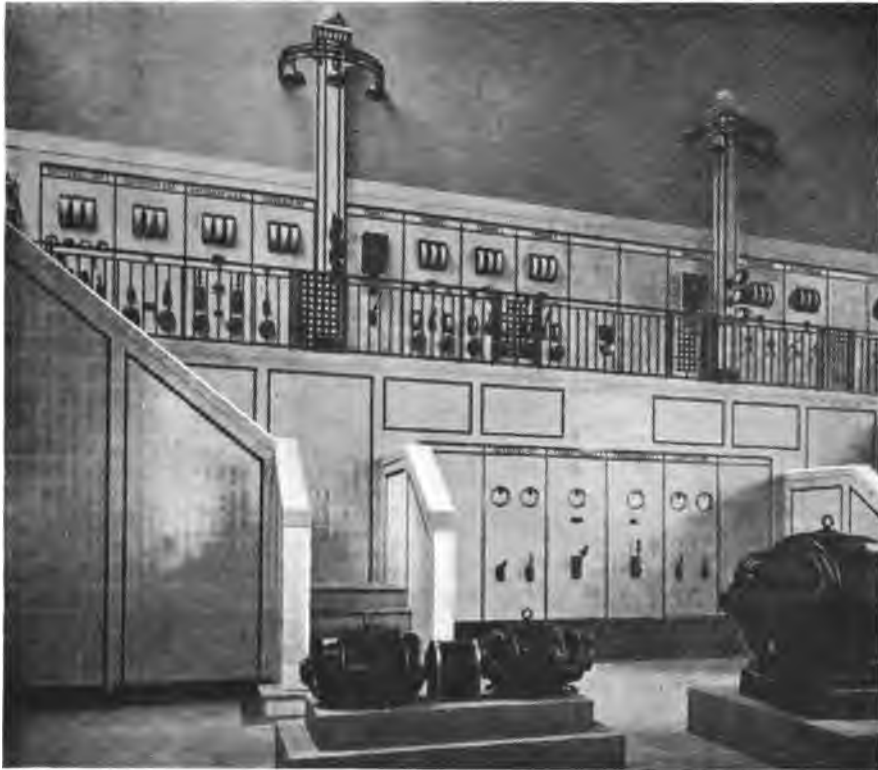
Fig. 37.—Operating Switchboard in the Electricity Works of the Hamburg Elevated Railway.
