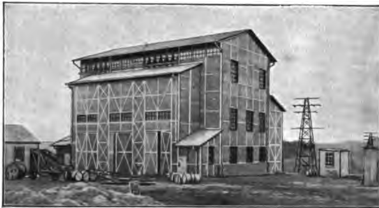
Fig. 151.—Bantjes Station (similar to Hercules Station). Main switch station for 40,000 and 20,000 volts, with transformer cells; in the background, masts for two 40,000-volt three-phase circuits with brackets for carrying three guard wires
