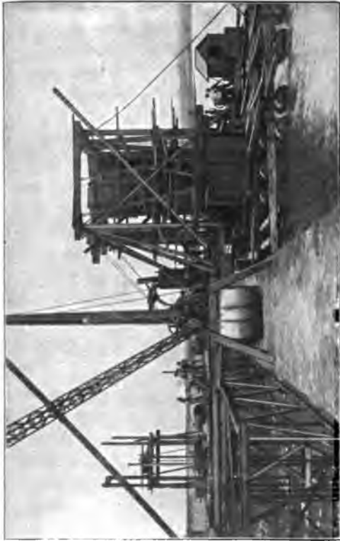
Fig. 129.—Rosherville Power Station Pumping Plant. To the right of the Dam, lowering a Caisson from a Raft; to the left of the Dam, Iron Framework for supporting the Caissons and Delivery Pipes.
