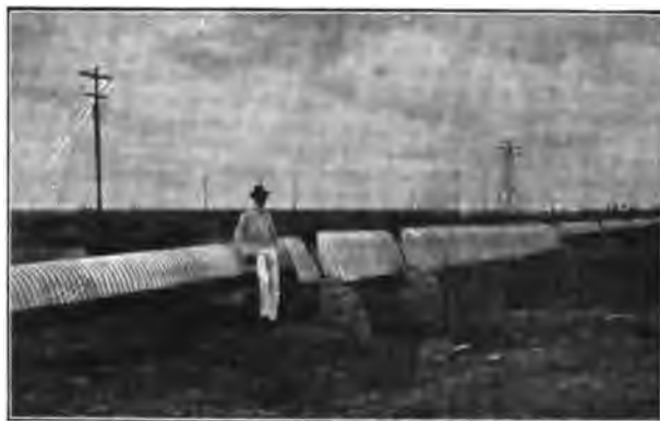
Fig. 160.--Compressed Air Plant. Compressed Air Pipe Line above ground, and covered with welded corrugated iron as a protection against the heat of the sun.
