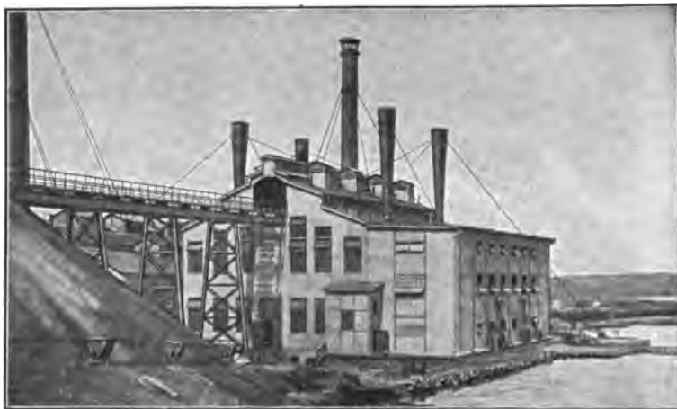
Fig. 101.—Brakpan Power Station.
