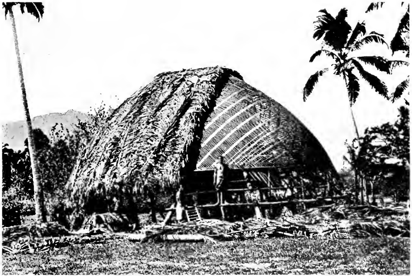
A SAMOAN HOUSE UNDER CONSTRUCTION
