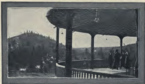
VIEW FROM THE MONTEZUMA BALCONY.
