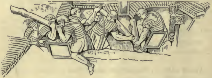
BUILDING A RAMPART
