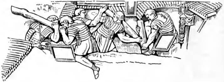
BUILDING A RAMPART
