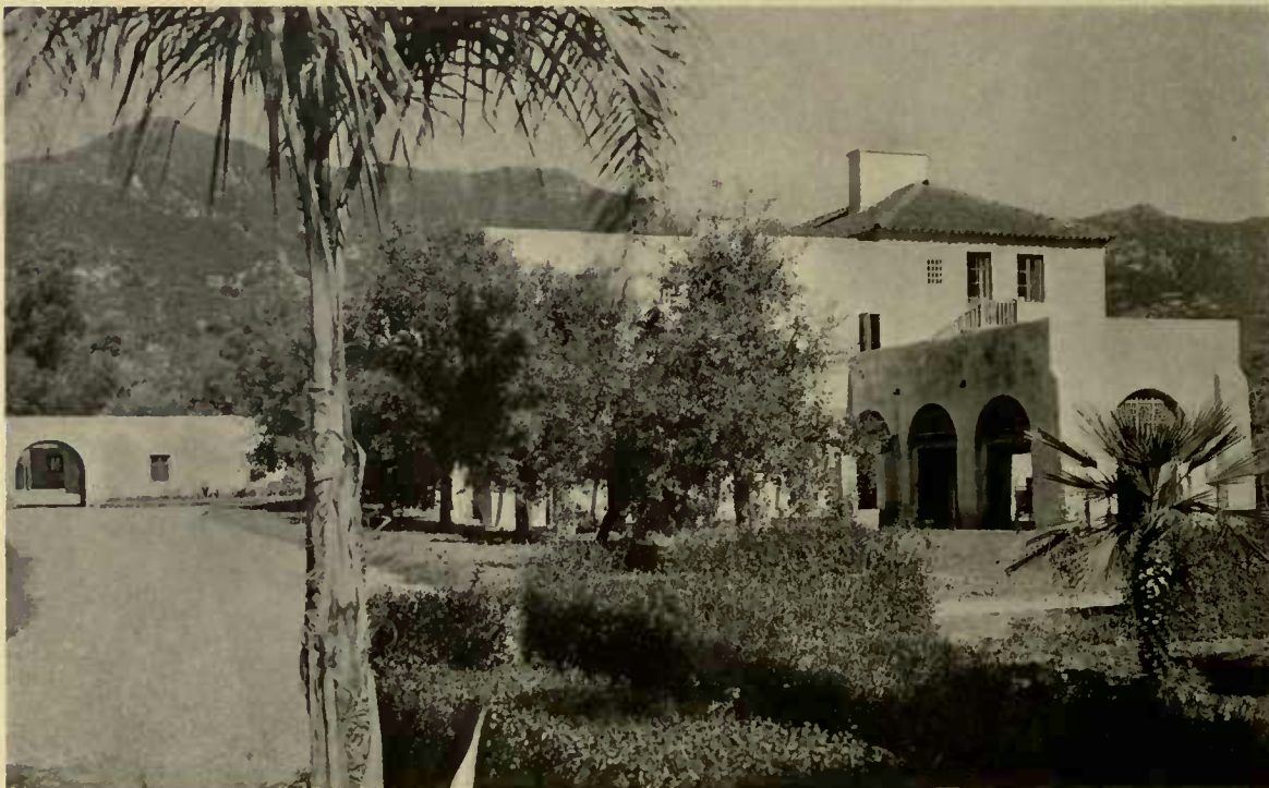
HENRY DATER HOUSE, MONTECITO, CALIFORNIA
