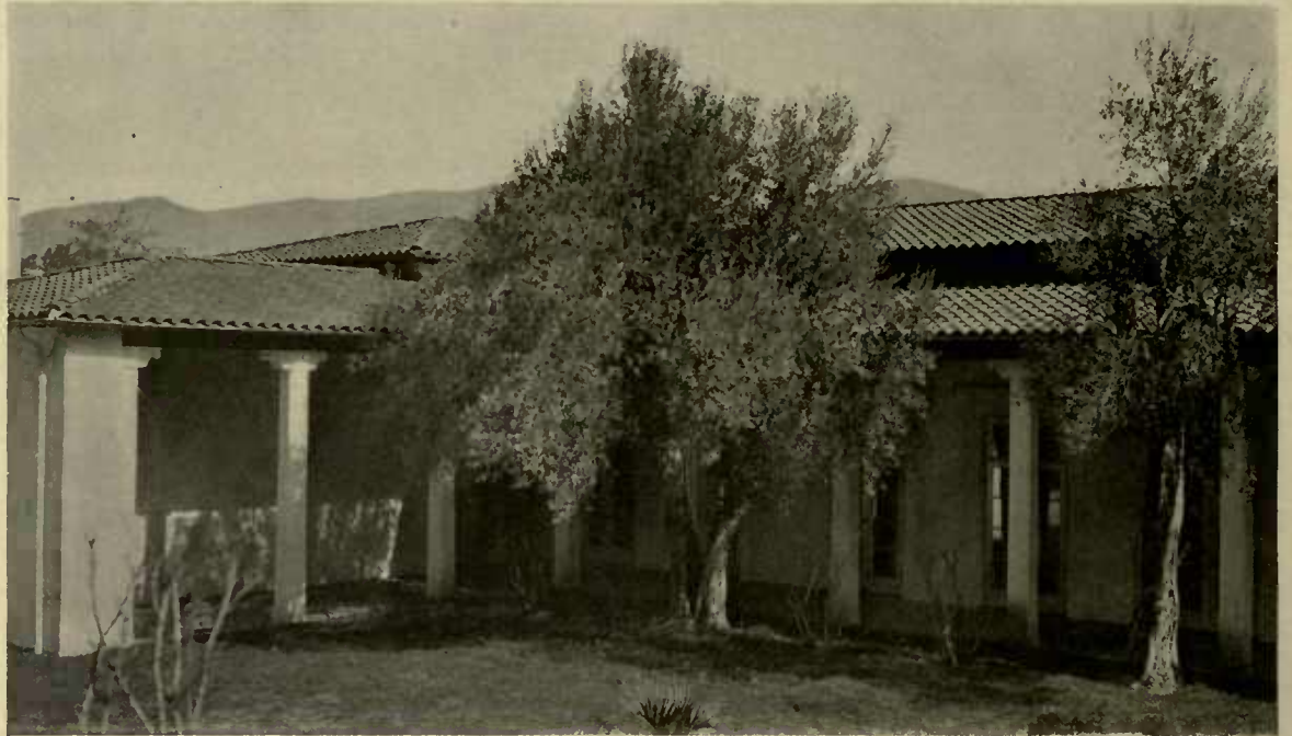
MAJOR J. H. H. PESHINE HOUSE, SANTA BARBARA, CALIFORNIA
