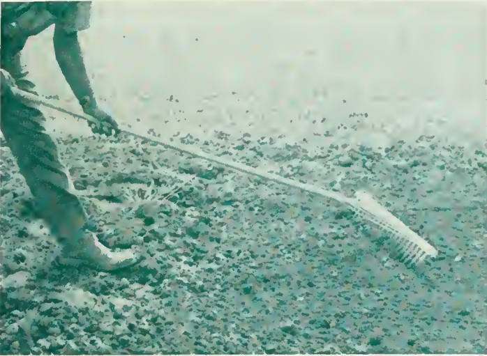
Preparing the final grade. (Fig. 3)
