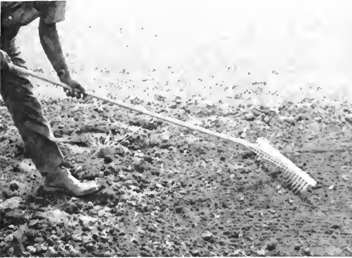
Preparing the final grade. (Fig. 3)
