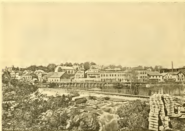
GREAT FALLS AND DAM FROM BERWICK SIDE.
