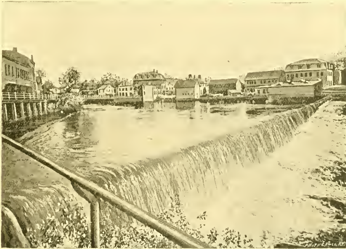
VIEW OF DAM FROM GREAT FALLS SIDE.
