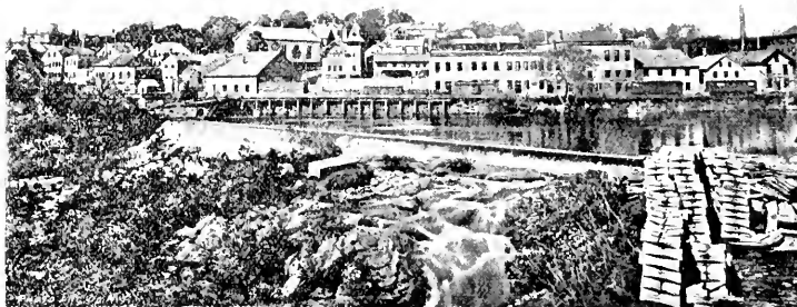
GREAT FALLS AND DAM FROM BERWICK SIDE.
