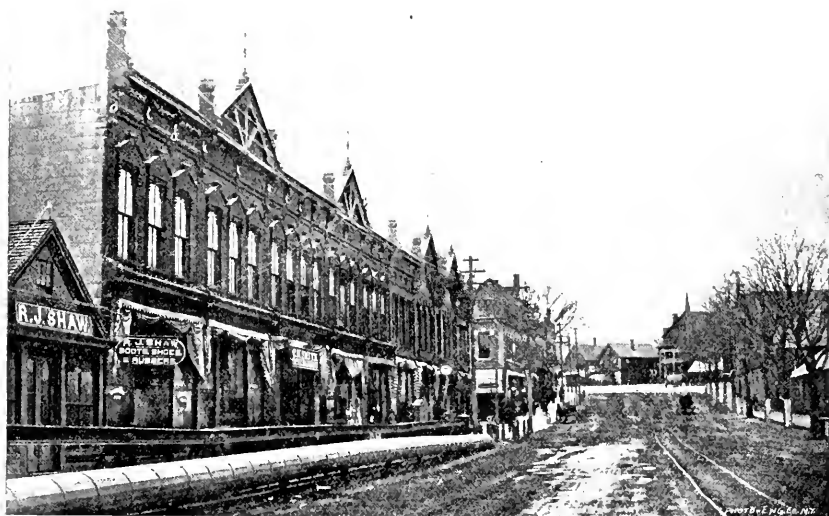
CENTRAL AVENUE, DOVER, LOOKING NORTH.
