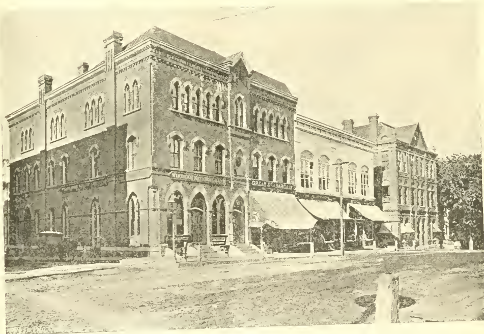
NORTH SIDE MAIN STREET, WILLIMANTIC, COR. BANK STREET.
