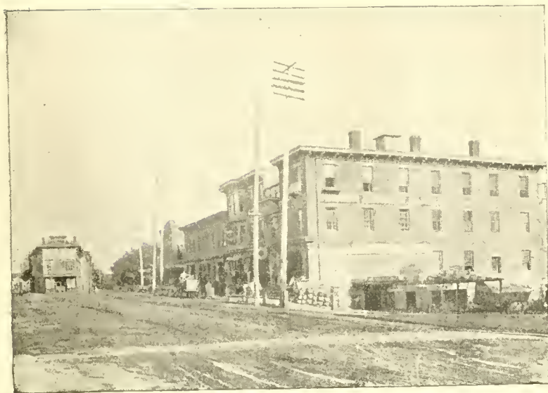
MAIN STREET COR. RAILROAD STREET.
