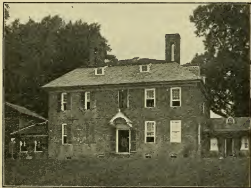
The Murray House, Anne Arundel County, Maryland Built in 1743
