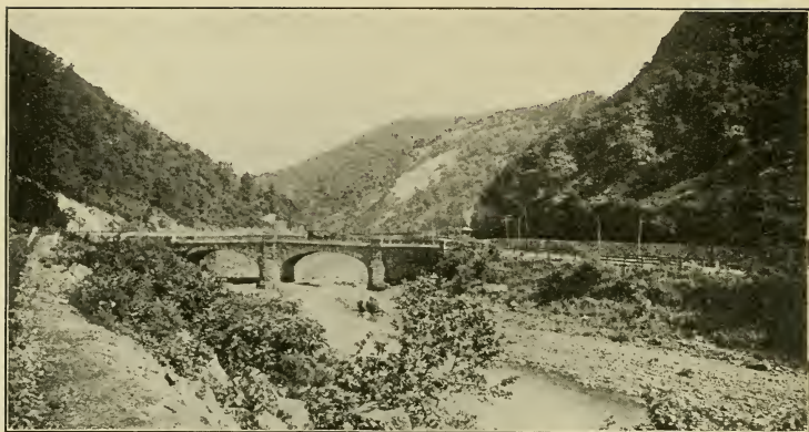
Old National Bridge, Cumberland
