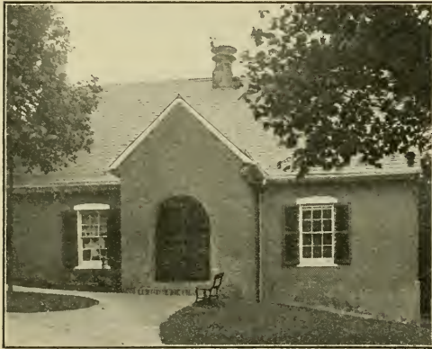
The Old Treasury Building, Annapolis 1
