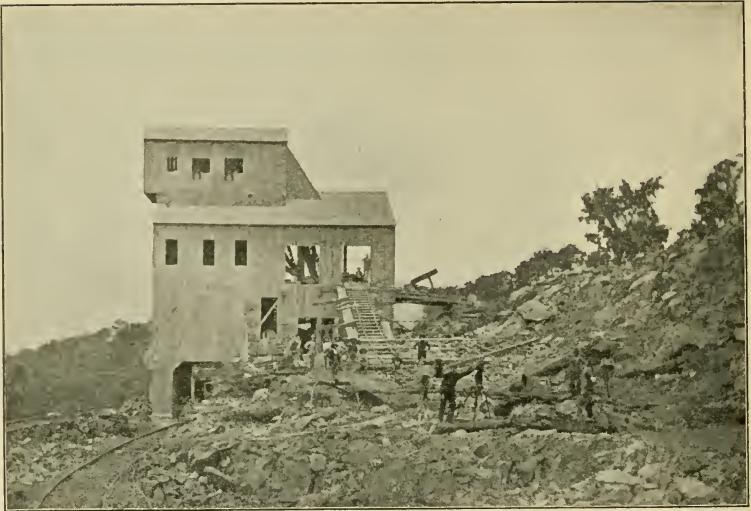
Limestone Crusher From a photograph
