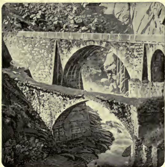
THE DEVIL'S BRIDGE.
