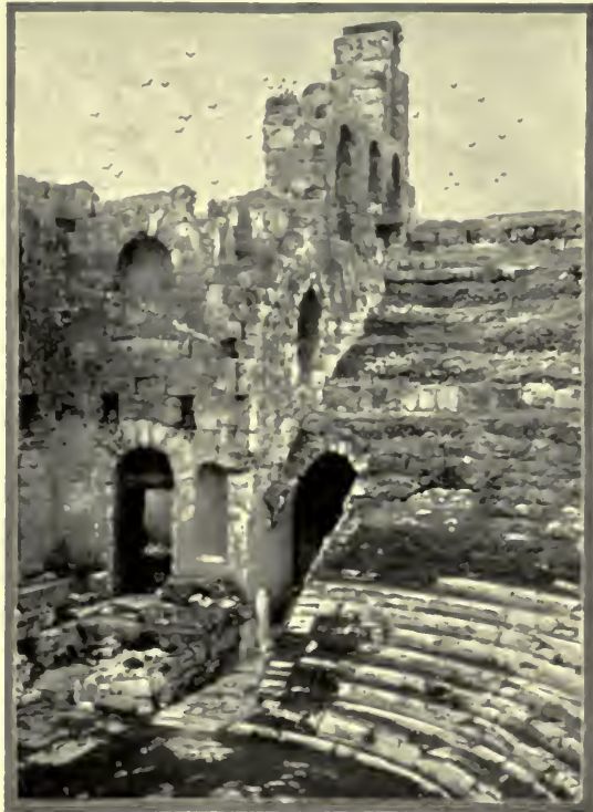
INTERIOR OF THE ODEON.
