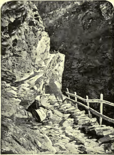
A FRAIL PARAPET.
