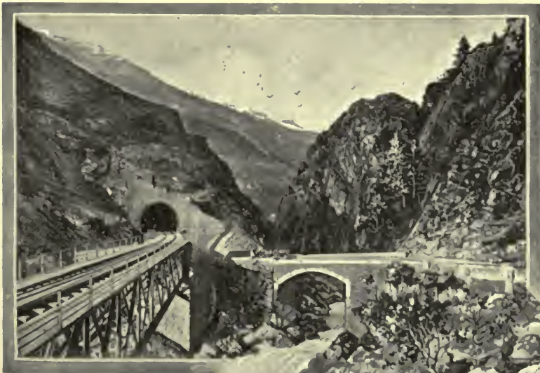
A PORTION OF THE ST. GOTTHARD.
