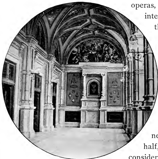
THE LOGGIA OF THE OPERA HOUSE.
