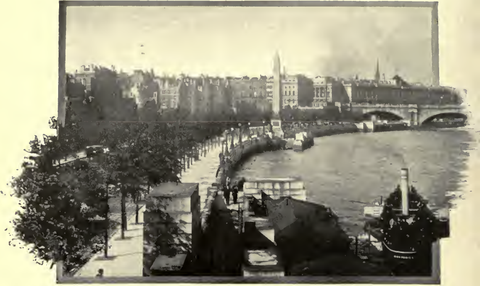
THE VICTORIA EMBANKMENT.
