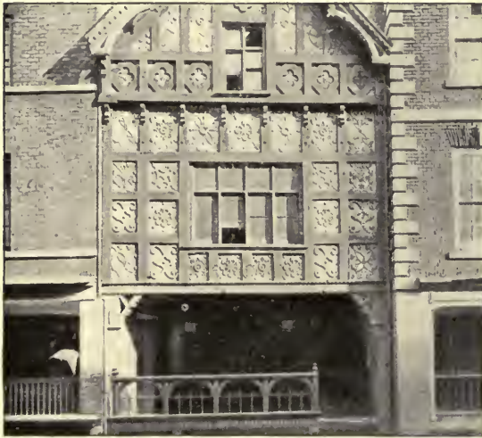
THE "RECONSTRUCTED" HOUSE.
