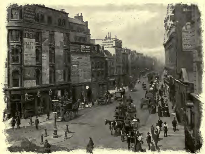
TOTTENHAM COURT ROAD.
