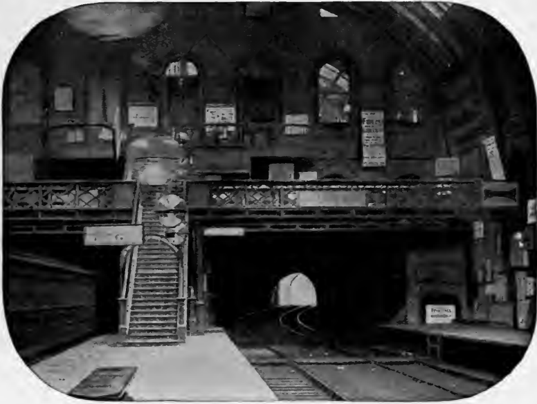
AN UNDERGROUND STATION.
