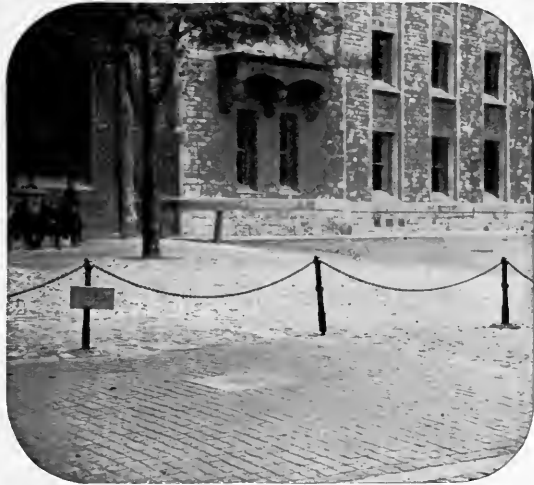
THE SITE OF THE SCAFFOLD.
