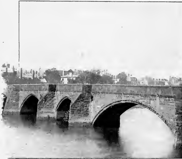
OLD BRIDGE AT CHESTER.
