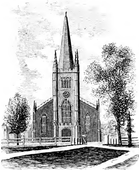
MEETING-HOUSE ERECTED BY THE FIRST PARISH IN 1833.
