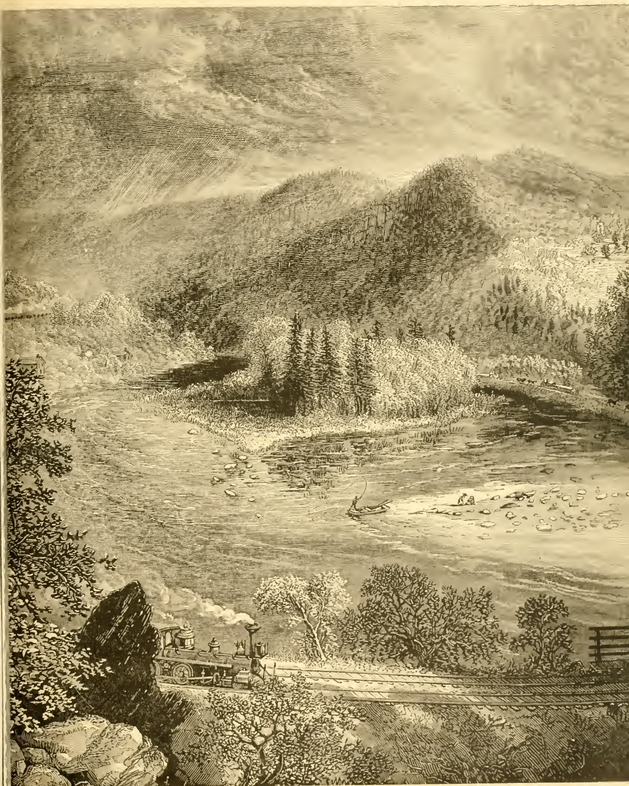
ROCK RIFT ON THE DELAWARE DIVISION ERIE RAILWAY, NEAR PORT JERVIS, N. Y.
