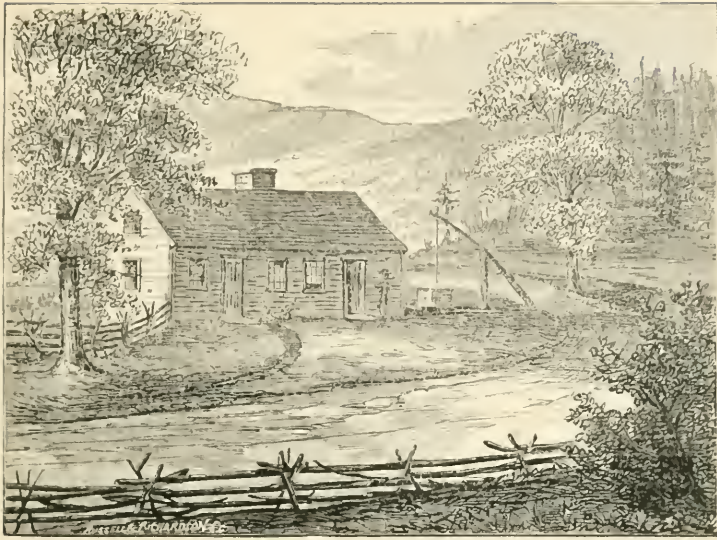
HOUSE IN LEOMINSTER.
